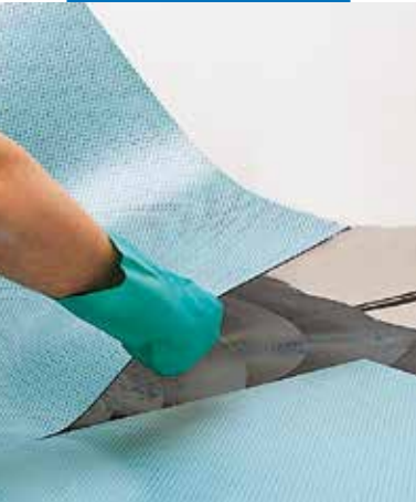
Laying conductive PVC tiles
