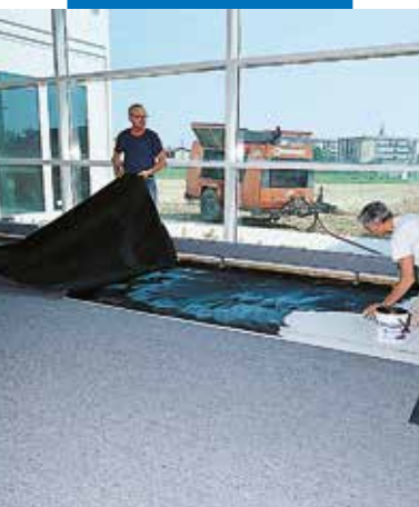
Installing industrial flooring in an electronics company
