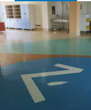
Example of PVC laid in a long-stay ward - San Martino Rest Home - Italy
