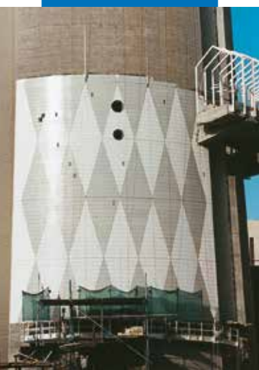
An example of an installation of klinker on concrete with Kerabond + Isolastic - New Telecommunication Tower - Kuwait City (Kuwait)
