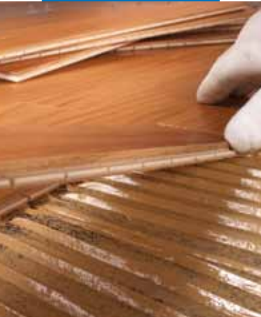
Laying small pieces of pre-finished parquet
