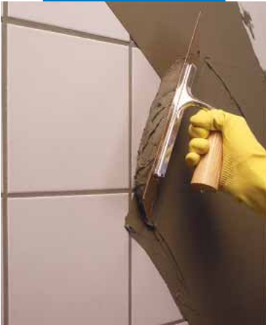
Smoothing an existing wall covering with Planipatch
