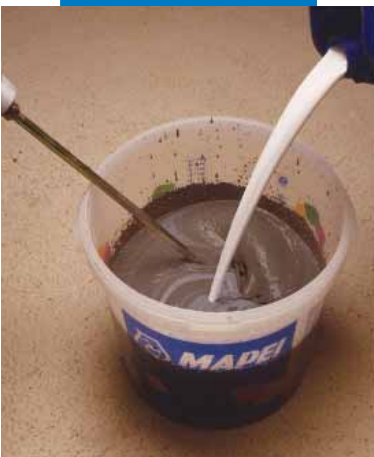
Mixing Planipatch with Latex Plus for smoothing difficult and deformable substrates
