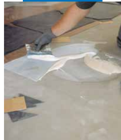
An example of an installation of inlaid PVC on a surface levelled with Ultraplan - CD 2 - Milan - Italy
