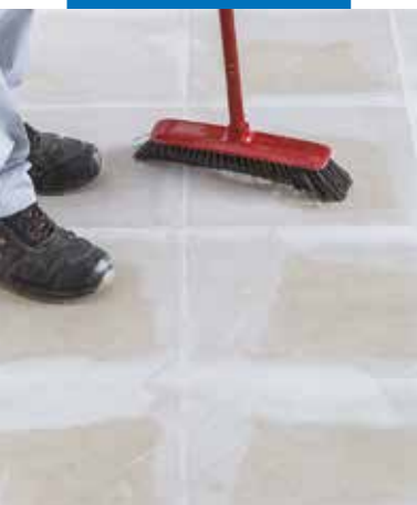
Removing dust after the sanding operation
