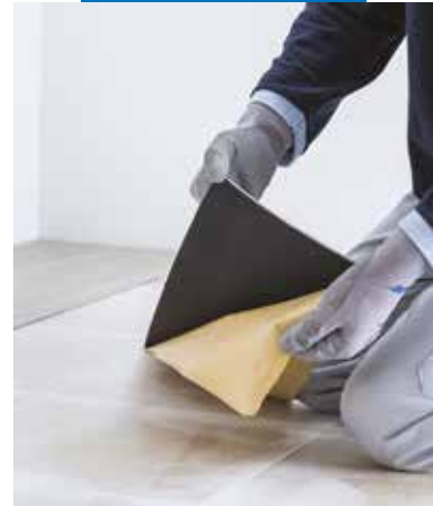
Removing the protective backing from self-adhesive LVT
