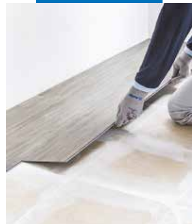
Laying click-connecting LVT over ceramic levelled off with Planiprep 4 LVT
