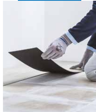
Laying self-adhesive LVT over ceramic levelled off with Planiprep 4 LVT
