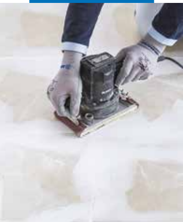
Sanding over the surface levelled off with Planiprep 4 LVT
