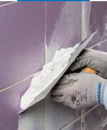
Levelling off of an existing ceramic wall with Planiprep 4 LVT
