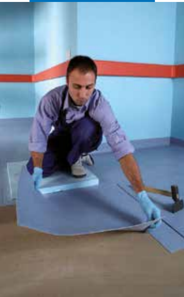
Installing PVC floor tiles
