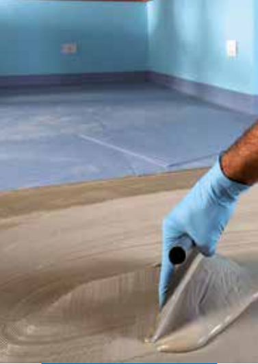
Applying Ultrabond Eco 380
