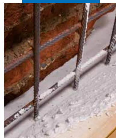
Close-up of Mape-Antique Colabile after pouring
