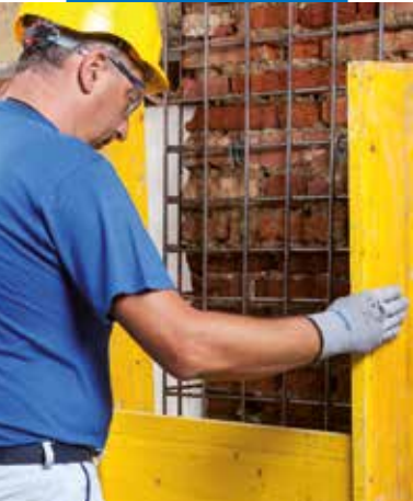
Placing formwork in position
