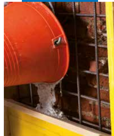
Pouring Mape-Antique Colabile into formwork
