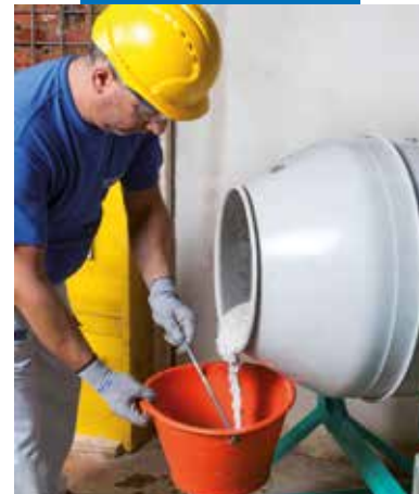
Pouring Mape-Antique Colabile into a bucket
