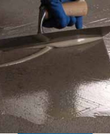
Priming the substrate
