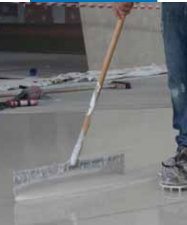
Application of self-levelling mortar
