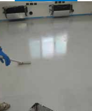
Finishing and waxing the surface
