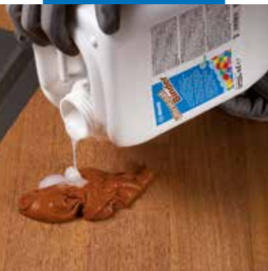
Mixing of Merbau powder with Ultracoat Binder
