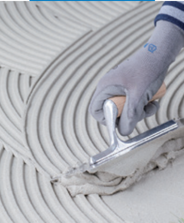
Spreading Adesilex P9 white
