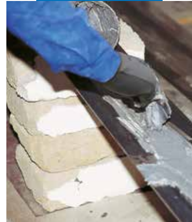
Application of Adesilex PG1 on metal sheet
