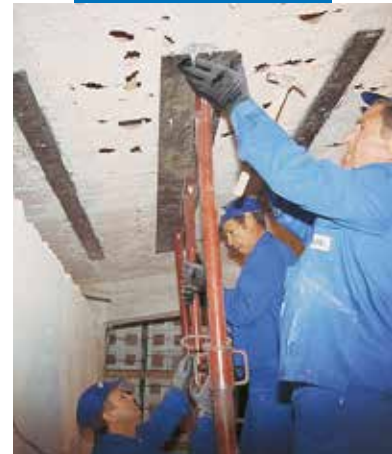
Placing metal sheet for structural reinforcement
