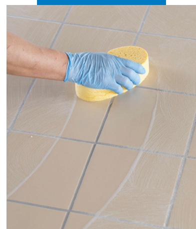
Cleaning and finishing joints with a hard cellulose sponge
