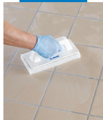
Cleaning joints with Scotch-Brite®
