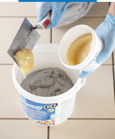
Pour the hardener (component B) in the container of component A
