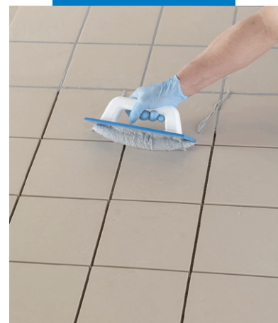
Application of Kerapoxy CQ with Mapei rubber trowel
