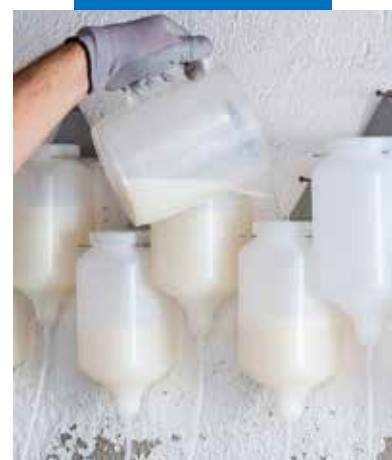
Pouring the mixture into the diffuser cups
