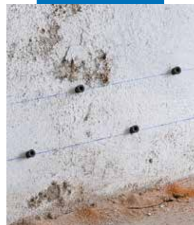
Detail of the staggered rows of holes
