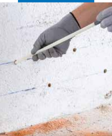
Inserting the injectors in the holes
