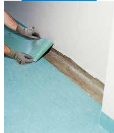
Installing PVCA flanking strip
