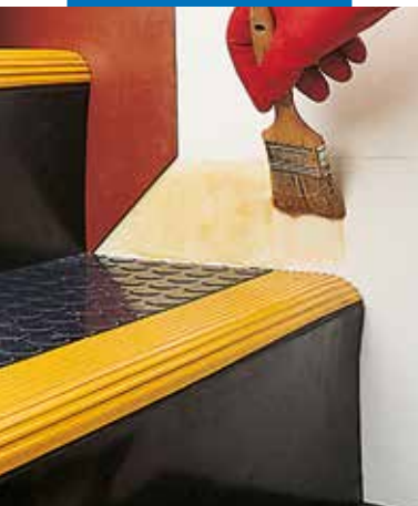
Installing rubber skirting with Adesilex LP
