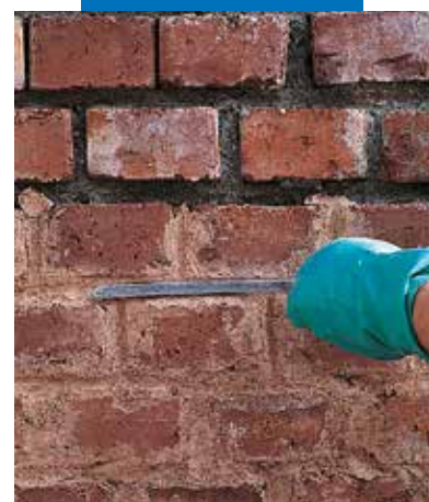
Finishing the joints pointed with Mape-Antique CC
