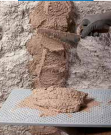
Preparation of levelling strips
