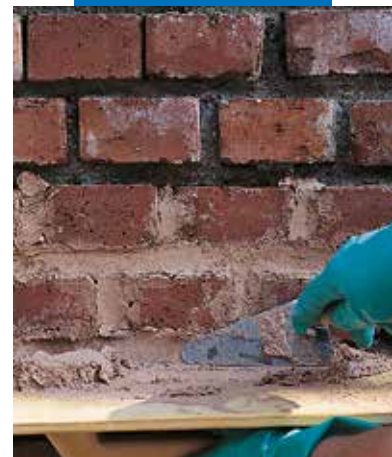
Pointing a brick work using Mape-Antique CC
