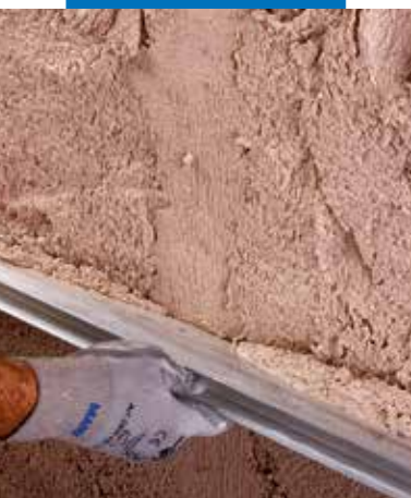
Flattening the surface of Mape-Antique CC with a straight edge
