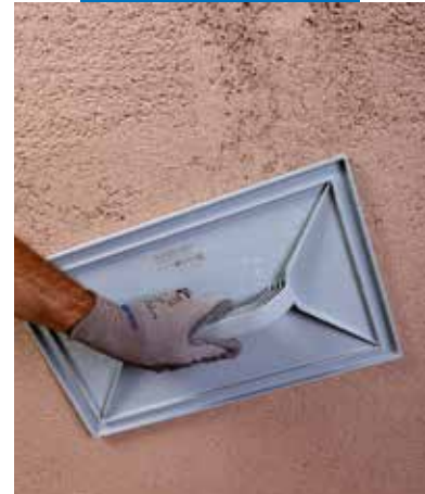
Levelling the surface of Mape-Antique CC
