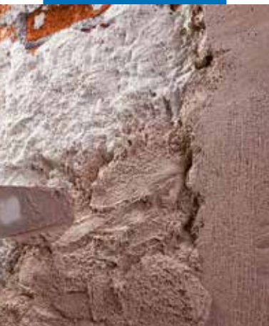
Application of Mape-Antique CC over Mape-Antique Rinzafo
