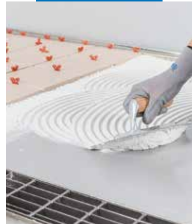
Applying the floor or wall covering with Kerapoxy Design
