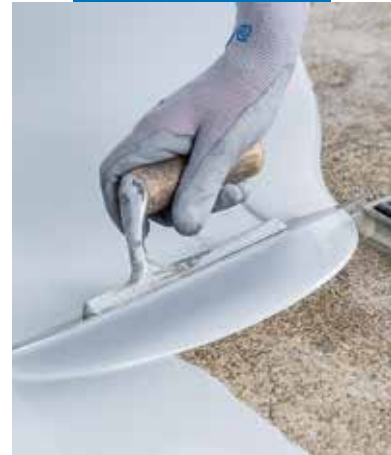
Application of Mapegum EPX
