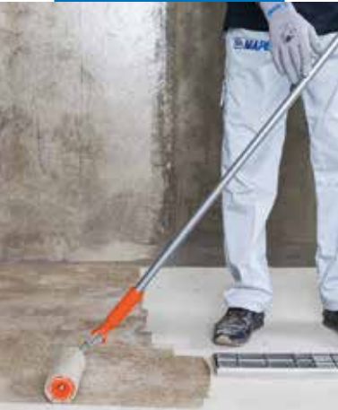
Application of Primer SN on the substrate
