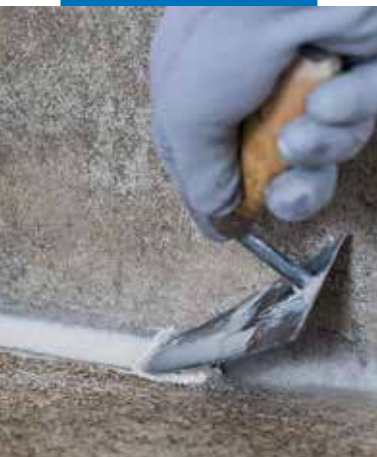
Forming fillet joints
