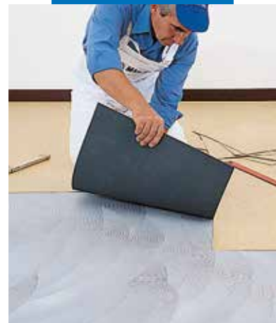
Homogeneous PVC installation
