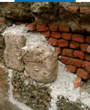
De-humidifying render rebuilding a wall using mortar on site
