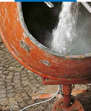
Mixing mortar on site with locally-sourced aggregates
