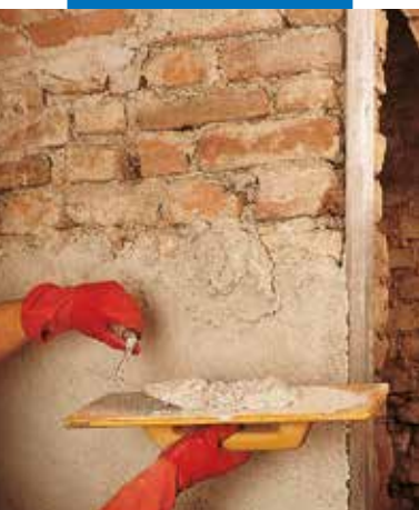
Application of de-humidifying render mixed on site
