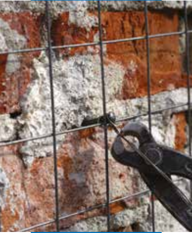
Fastening zinc-plated mesh to the masonry
