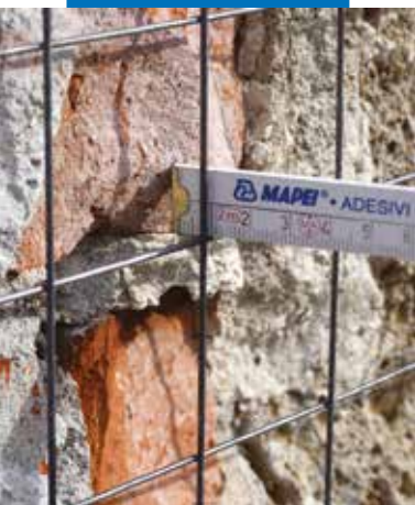
Checking the gap between the mesh and substrate
